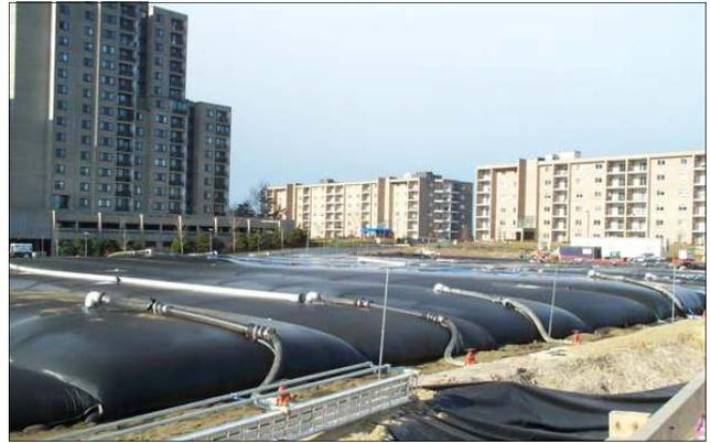
Impacted sediments from the Geotube® containers were blended with on-site soils and imported fill. More than 100,000 cubic yards of soils and sediments were mixed on-site and spread as backfill to achieve pre-construction grade.
