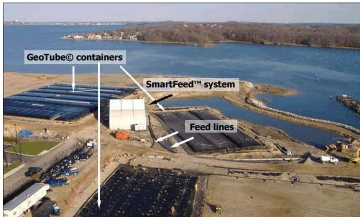
A temporary building was erected to enclose the SmartFeed™ system. The SmartFeed™ system filtered and treated the hydraulically dredged sediments at a rate of 3,500 gpm.
